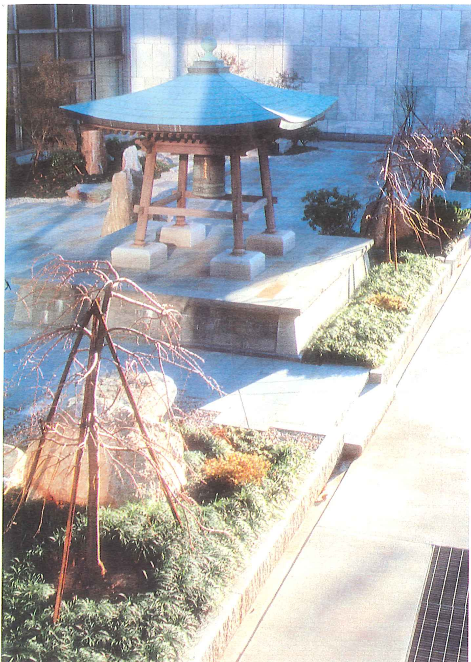
Pennsylvania Bluestone and Chelmsford granite were both employed for the bell tower base. Pennsylvania Bluestone makes up the top and sides of the base, with Chelmsford granite employed for the base blocks and cornerstones.
