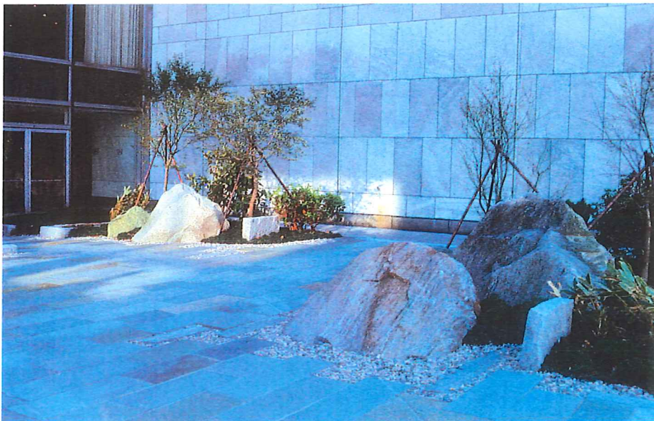
Bluestone was employed as pavers for the garden floor. The material worked well for the floor because of its slip-resistant qualities, according to Abe. The stone was also selected for its natural beauty and unique color patterns, with pieces tending toward gray, blue or red in color.
